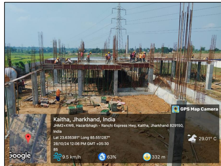
Main building under Construction
