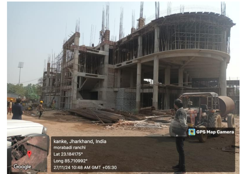
State Library under Construction
